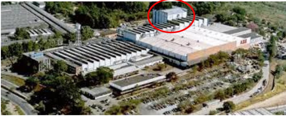
ABB Power Transformer factory, Guarulhos - highlighted is building home to one of the world's largest Van de Graaff Generator's used to test transformers for lightning strikes.
